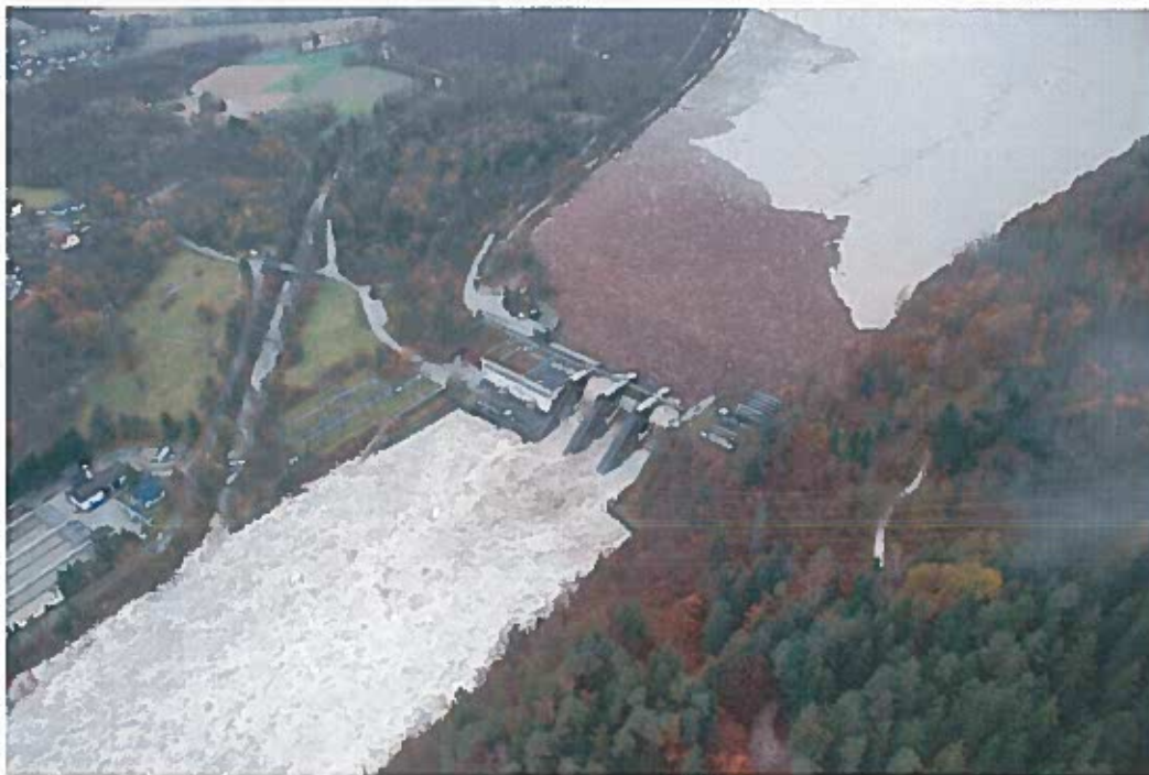
Photo 8: Draa at hydrological power plant Ferlach (Verbund AG)
